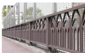
高欄 Bridge railings
