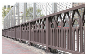
高欄 Bridge railings
